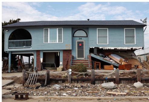
After Superstorm Sandy, LEHMUA relied on the FlexNet network to prioritize relief efforts and quickly restore service to the devastated area.
